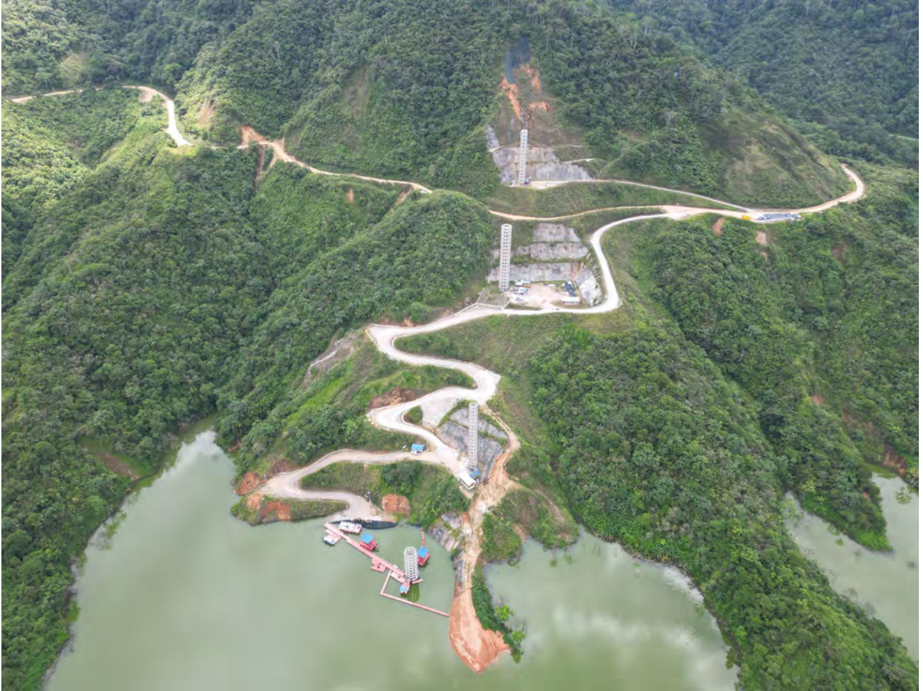
Mirador Tundayme tailings dam is planned to be tallest in the world 1050 feet high with no emergency response plan
